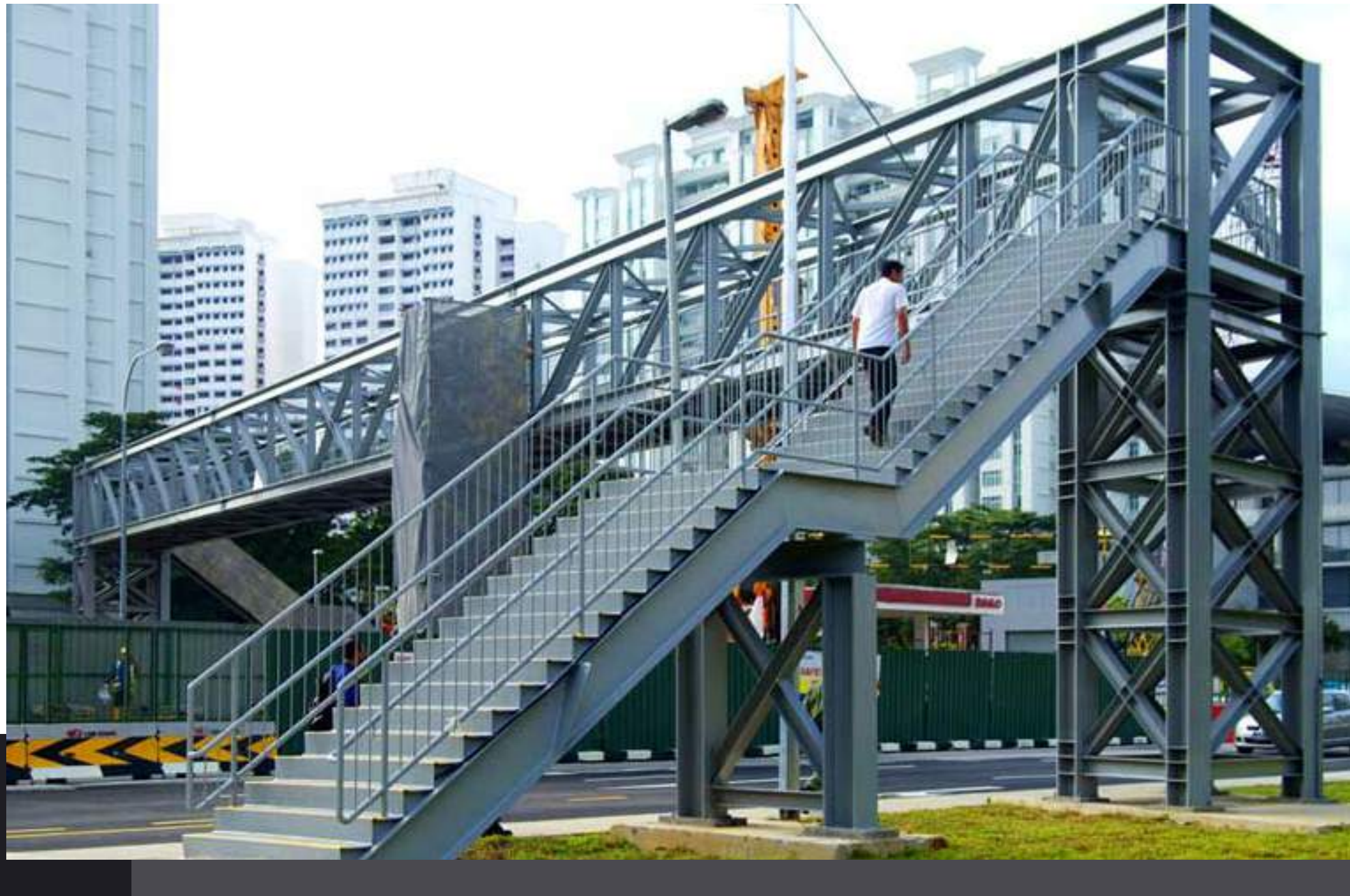
IRON PADESTAL BRIDGE
